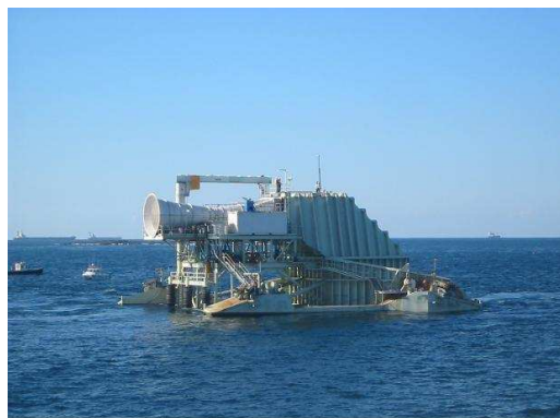
Figura 2.4: Central Energetech - Vista lateral.
